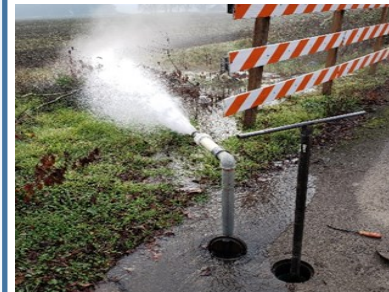
Pacific Lumber New Fire Suppression System Line
