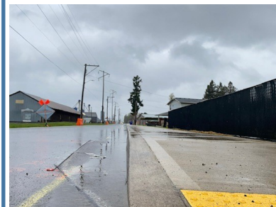
Matthieu St. Improvement Project
