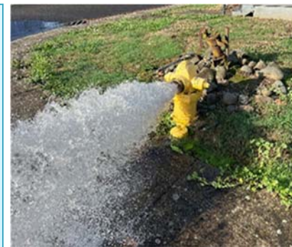
Distribution System Flushing
