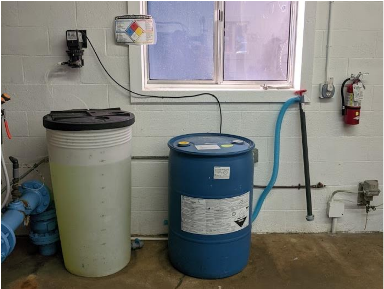
Figure V-3. Existing Sodium Hypochlorite Feed System
