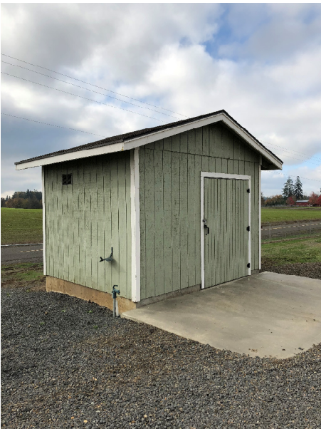
Irrigation Pump Station Building
